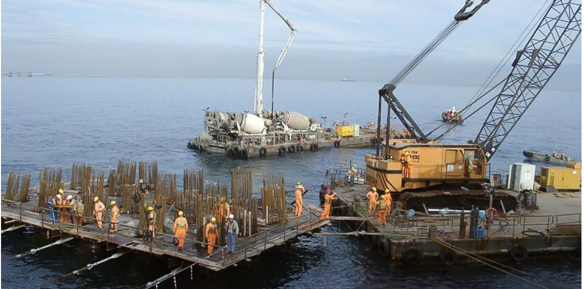
Figure(10) pum placing concrete
